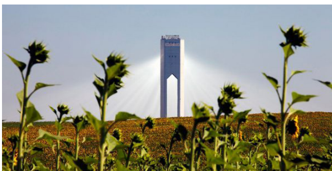
Typical CSP central receiver -power tower- technology.
