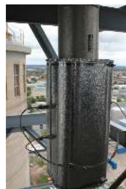
An example of proper tracing and insulation of a diaphragm
