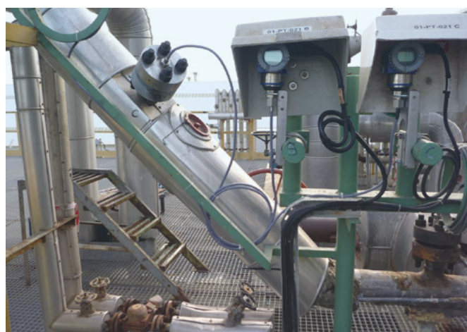
Pictures of installation of the diaphragm seal systems that experienced frequent failures at Profertil's Bahia Blanca site.
