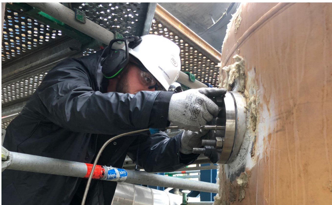
Turnaround dismantling activities of diaphragm seals in full swing. In total 18 instruments were checked, repaired or delivered new.
