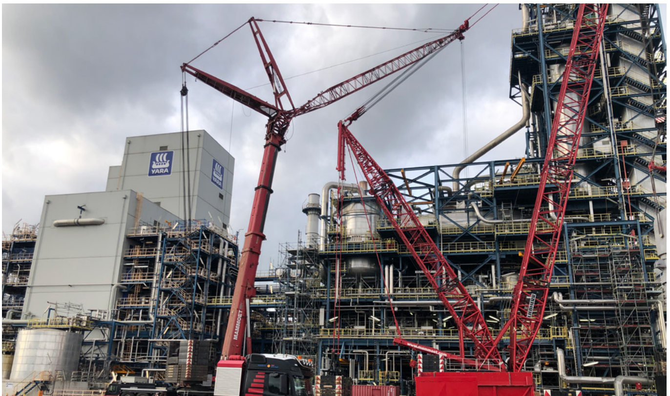
Turnaround activities underway at Yara International's production site in Sluiskil, The Netherlands.
